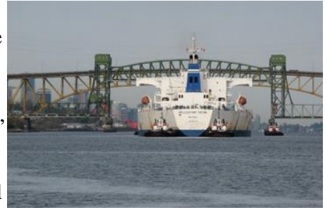
AFRAMAX FREIGHTER APPROACHING RAILWAY BRIDGE AT SECOND NARROWS Source: BCWaters.org
