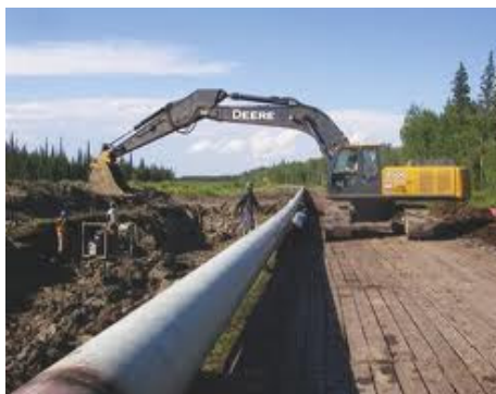
Source: Pipeline International PIPELINE CONSTRUCTION IN ALBERTA
