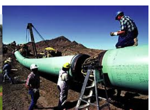
Source: Oil and Gas Journal TRANSCANADA PIPELINE LTD. CONSTRUCTION
