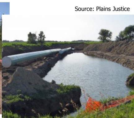
Source: Plains Justice KEYSTONE PIPELINE NEAR YANSTON, SD
