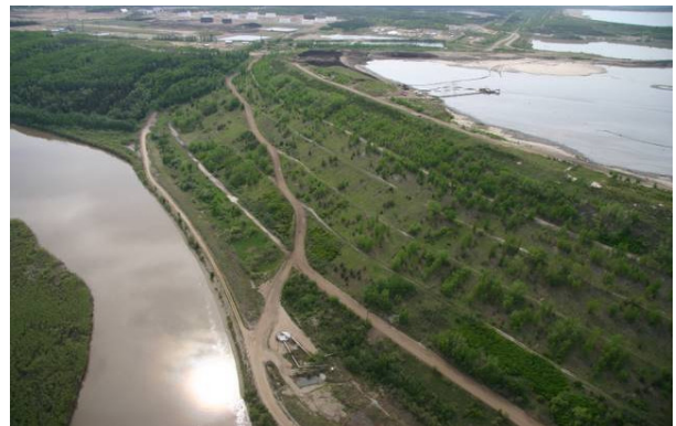
"...Tar Island Pond One, situated right on the banks of the [Athabasca] river, built 300 feet high above the river. It leaks 67 litres of toxic tailings water per second." Water expert, Dr. Kevin Timoney [6] Photo: David Dodge, Pembina Institute
