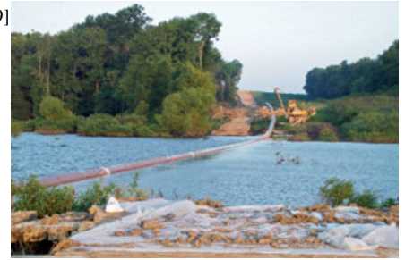
KEYSTONE PIPELINE WATER CROSSING IN THE MIDWEST Source: North American Pipelines
