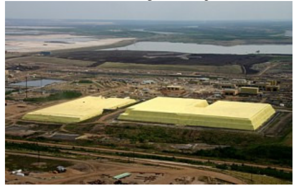
SYNCRUDE SULPHUR STORAGE AT PROCESSING FACILITIES
